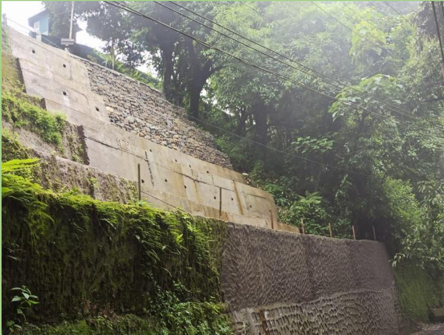
Restoration of landside near office area
