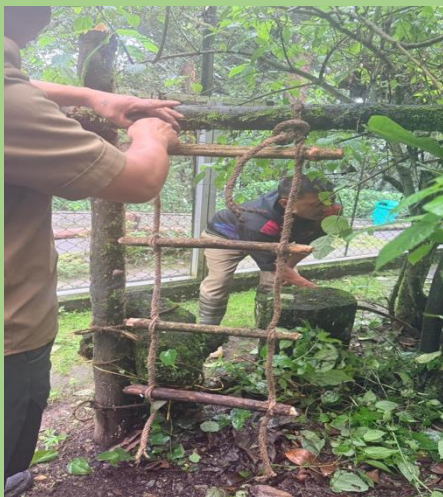
Installation of ladder at Asian Palm Civet enclosure
